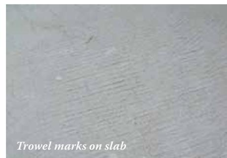
off. Further investigation revealed that the GC gave up and walked away from final finishing of the slab after waiting 17 hours for steady rainfall to stop, which didn't happen that night. They ended up grinding 1/2" off the subfloor during the quality assurance flooring program that was in place for that project.
